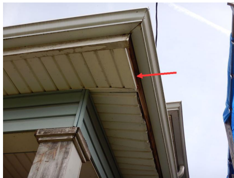
Opening at roof edge
